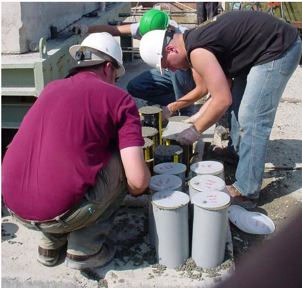
**Figure 3.15 – Strength and shrinkage molds cast during trips to precast yard.**
