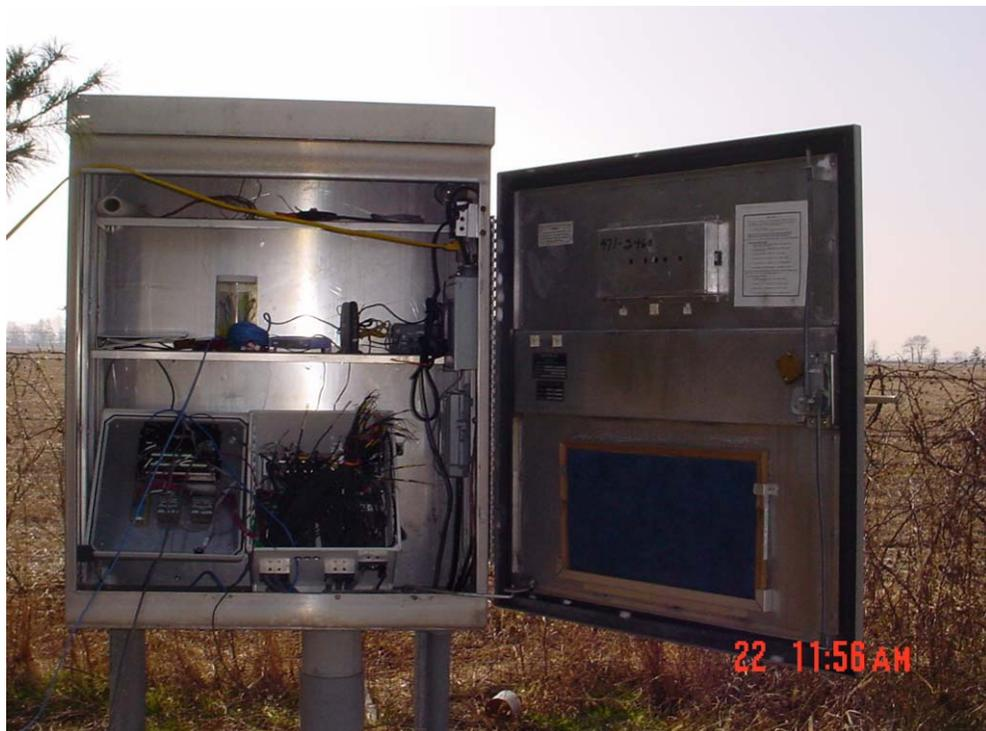
**Figure 3.14 – Signal cabinet with main data-acquisition equipment installed at the edge of right of way.**
